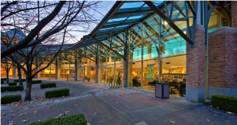
Figure A2. Port Moody Public Library
