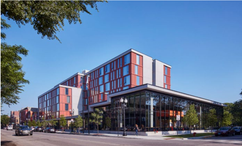
Figure A5. Taylor Street Apartments and Little Italy Branch Library, Chicago IL, SOM
